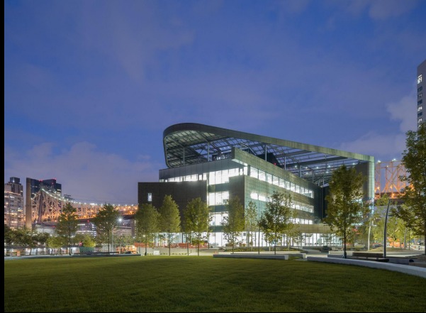
The Bloomberg Center is one of NYC's only buildings designed to be net-zero
